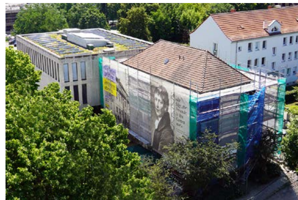
Renovation work on the old building of the Kleist-Museum, 2023 ©Stiftung Kleist-Museum
